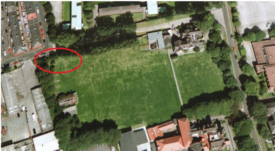
Aerial image from 2003 showing boundary trees in the north western edge of the site circled red
